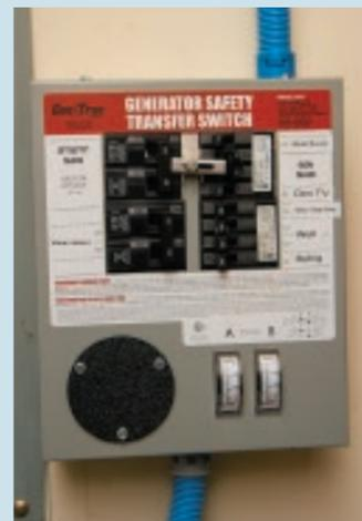
Have a licensed electrician install a transfer switch if you want to connect a generator directly to your home's electrical system. The switch prevents electricity from flowing back onto Walton EMC's electric system. An improperly connected generator can kill unsuspecting line technicians or anyone else who comes in contact with a downed line.
