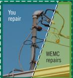
A service mast and weather head assembly connect to the inside wiring at this home.
