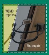
At this home, a house knob is used to attach WEMC's service wires. The wires enter a weather head and then go inside the home.
