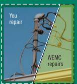
A service mast and weather head assembly connect to the inside wiring at this home.
