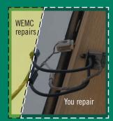
At this home, a house knob is used to attach WEMC's service wires. The wires enter a weather head and then go inside the home.
