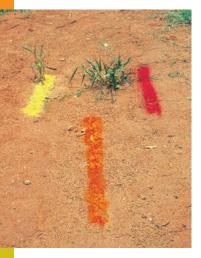
Ever wonder about paint marks like these on the ground? They show the location of underground utility lines. Each different line has its own identifying color. Electric lines are marked red, gas lines are marked yellow, telephone and cable are marked orange and water is marked blue. There are even more colors for other types of lines.
