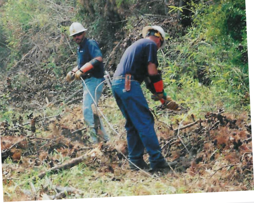
Above: Utility crew member Eric Ellington and Ronnie Browning pull fallen powerlines from debris along right-of-way in a deep forest before the lines could be reset. Photo and caption courtesy of Wayne Ford, Athens Banner-Herald, September 25, 2005.
